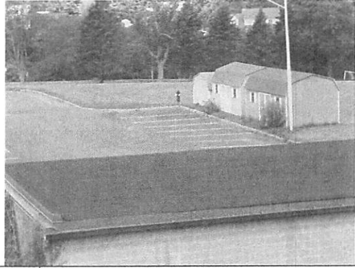
Photo #14: Garage area with modified roofing
