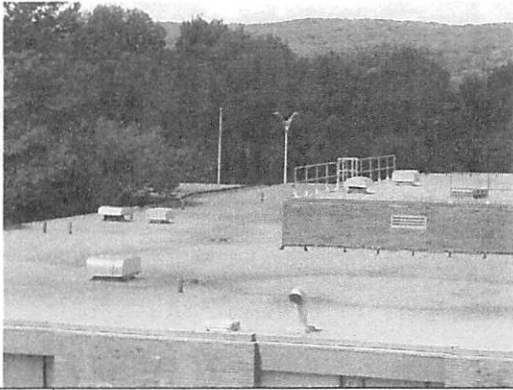
Photo #13: Overview of the 1998 sections
